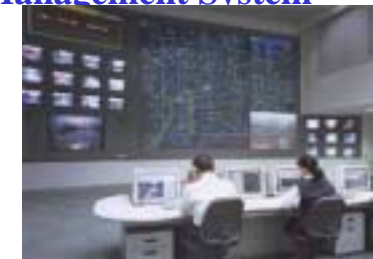
Traffic/Road Management System
