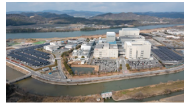
Left: No.1 Solar Power Plant Right: No.2 Solar Power Plant
